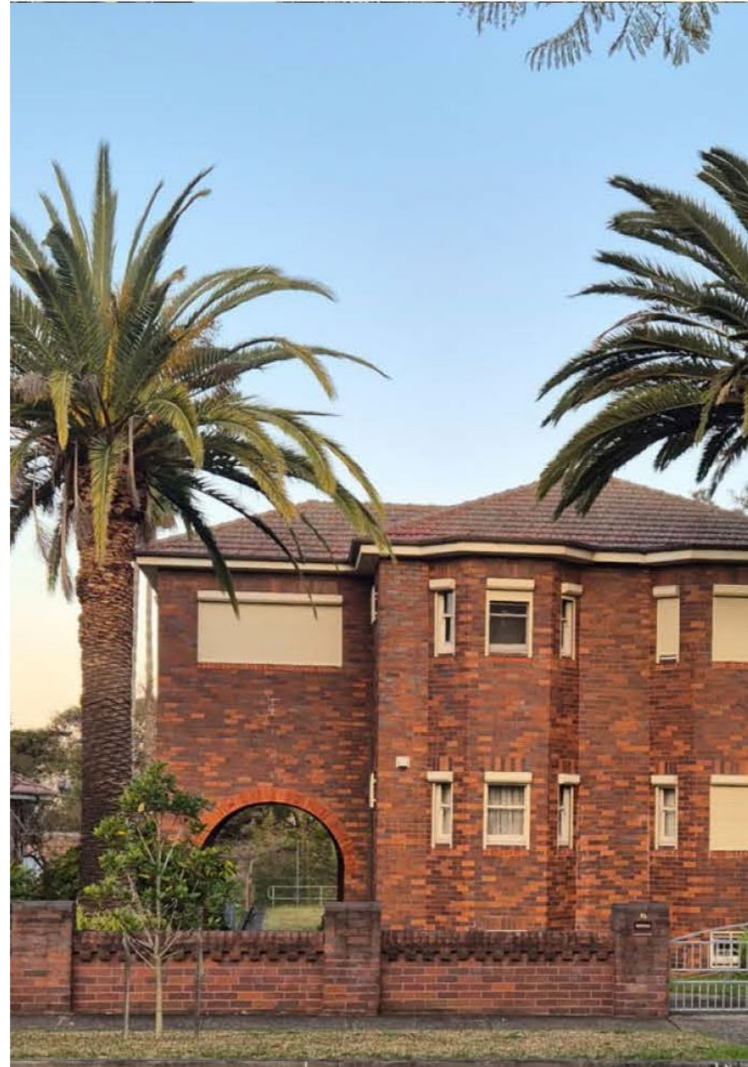
Figure 33. 18 Wallace Street, Burwood Source: TKD Architects
