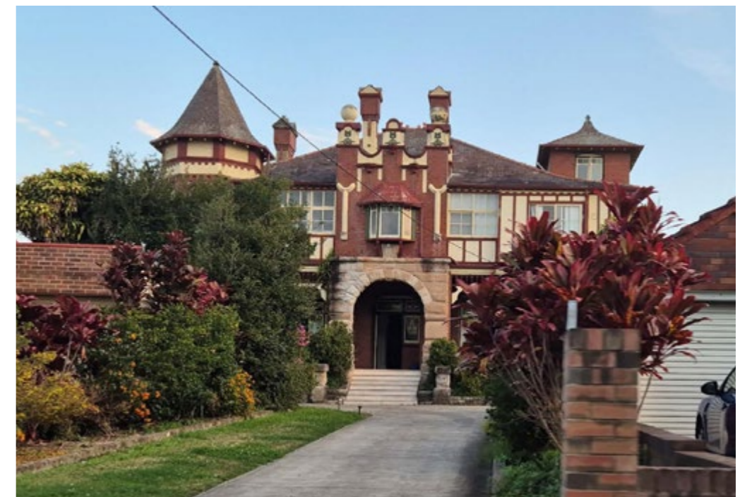
Figure 34. Heritage Item 13, 16 Brooklyn Street, Burwood Source: TKD Architects
