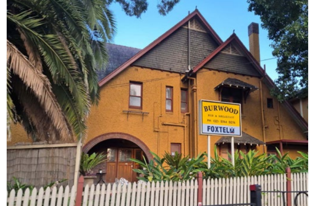
Figure 35. Heritage Item 108, 90 Shaftsbury Road, Burwood Source: TKD Architects
