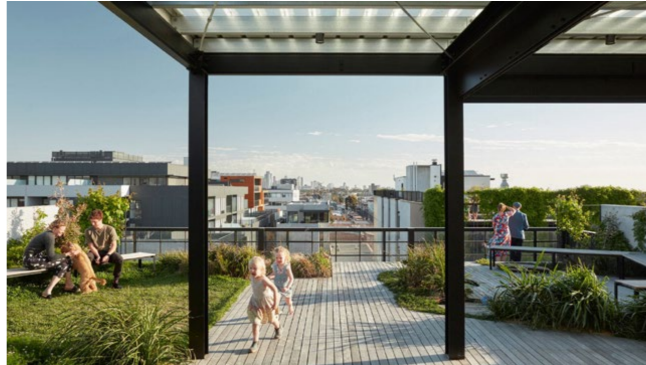
Figure 52. Rooftop garden at Nightingale 1. Design by Openwork and OCULUS. Source: Breathe Architecture
